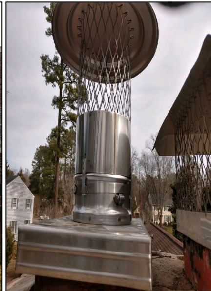
At the Rectory this week: Repairs to Rectory Chimney Oil Furnace Flue Liner & Cap
